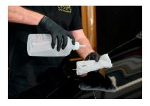
Note: No other cleaner (surface cleaner, etc.) may be used for the final surface pre-cleaning, as this can attack the adhesive on the CYS TPU and have a negative effect.
